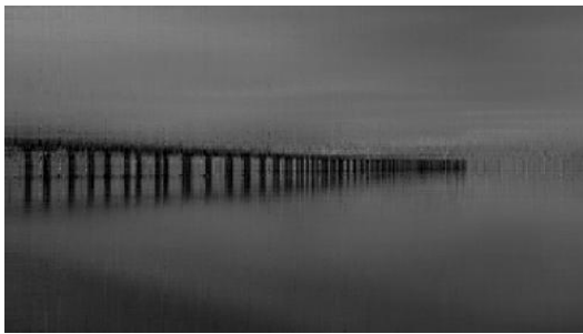
Bridge restored with CSNN-0.7
