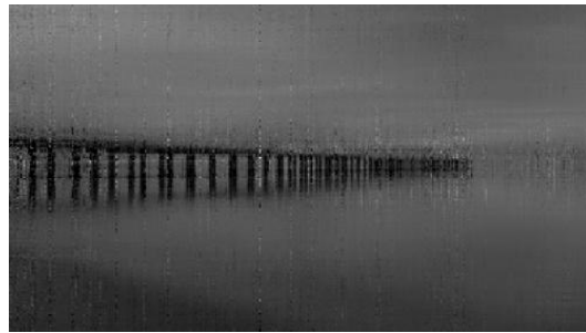
Bridge restored with CSNN-0.5
